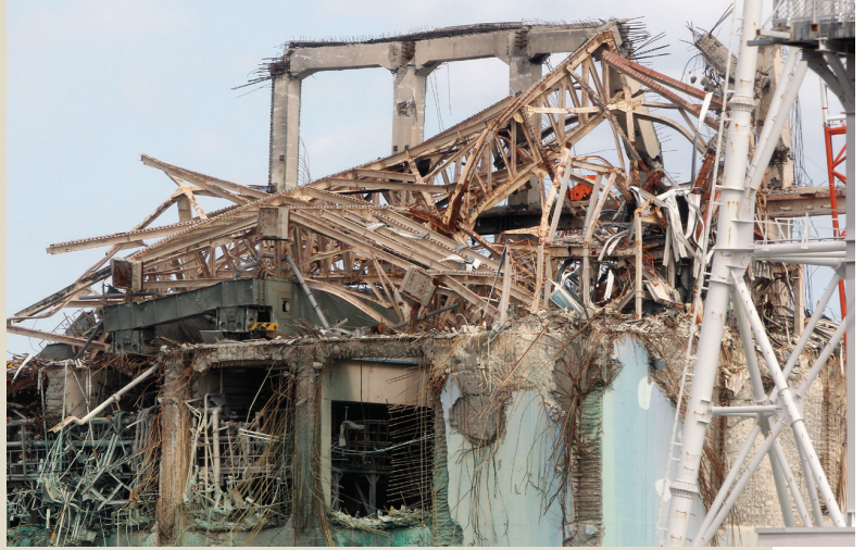
A damaged building at the Fukushima Daiichi nuclear power plant 1 year after the earthquake and tsunami
