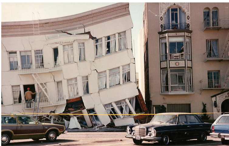
Damage to buildings in San Francisco after the 1989 Earthquake
